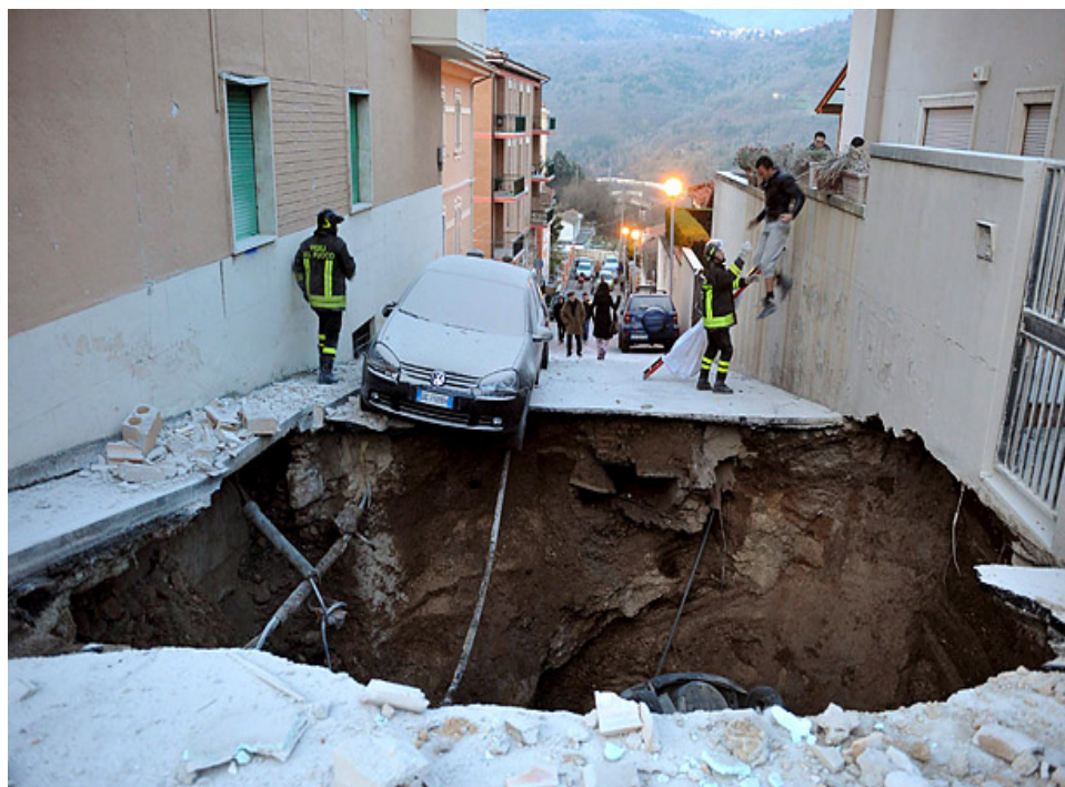
A street is damaged after Italy's worst earthquake in recent history in L'Aquila, Italy. Over 280 people died in the quake. –Time Magazine
